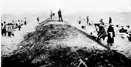
THE GREAT BUND BUILT TO KEEP BACK THE MARSH
